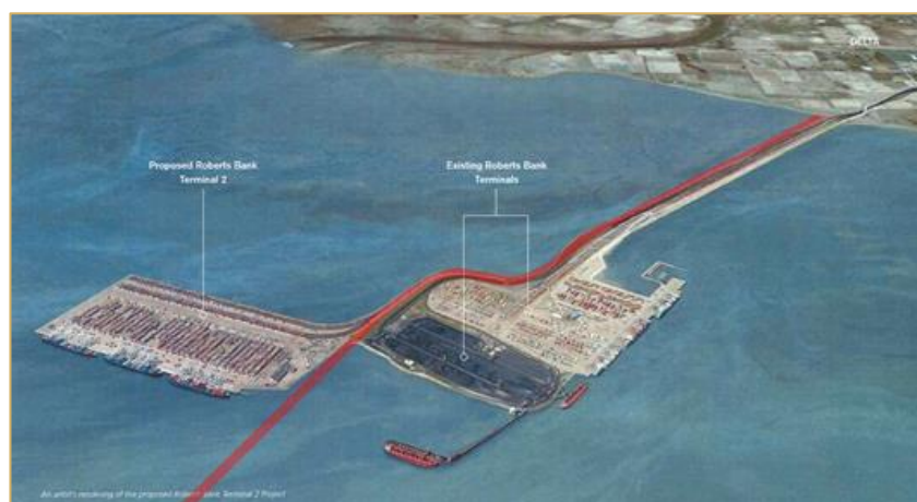
PHOTOGRAPH 1: ROBERTS BANK 2, BC, CANADA
